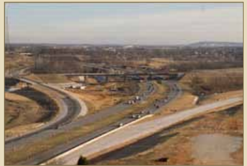
Perry Road Interchange
