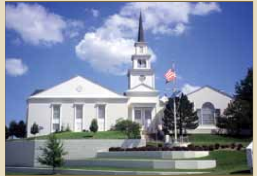
Kirk of the Hills Presbyterian Church Renovation
