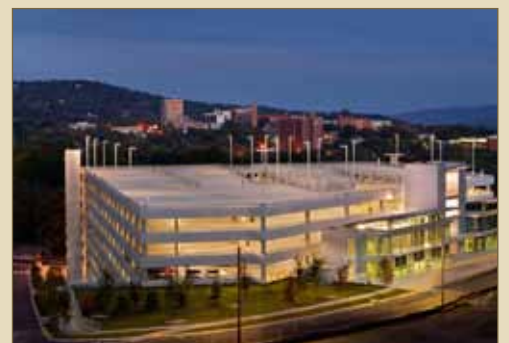
University of Arkansas Parking Deck
